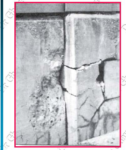
The concrete supporting a bridge has fractured.
