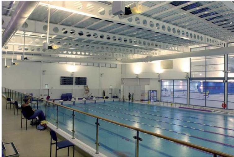
الشكل (11-9) Beams with circular web openings
