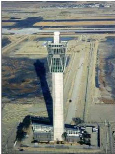
Air Traffic Control Tower: 100.4 m Natural Frequency: 0.71 Hz
