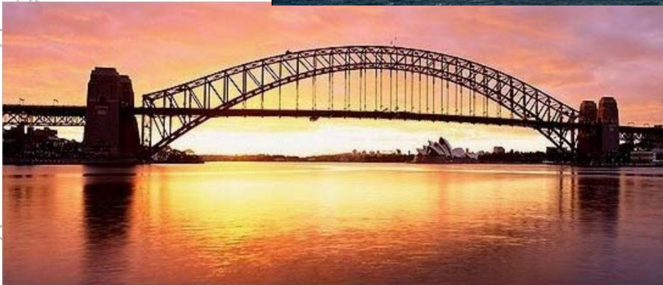
Sydney Harbor Arch Bridge
